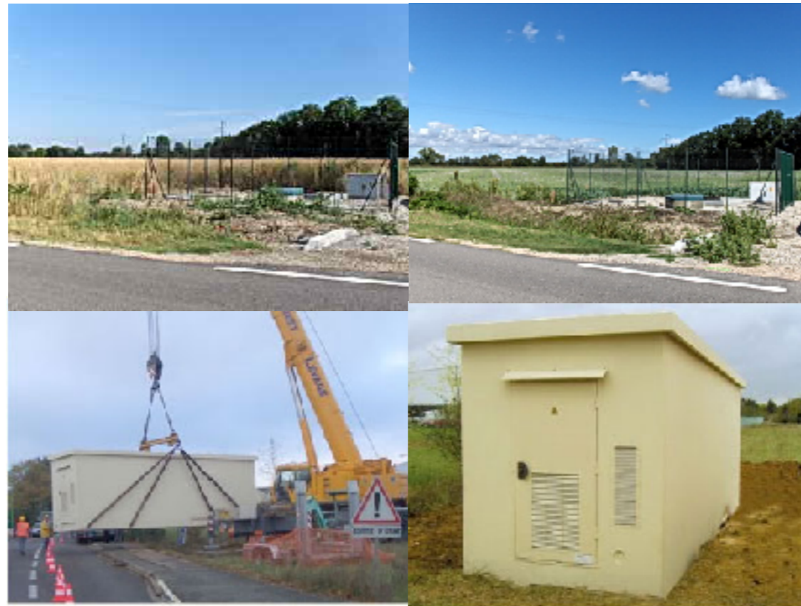
Deployment of a PoP of the Orange French backbone
